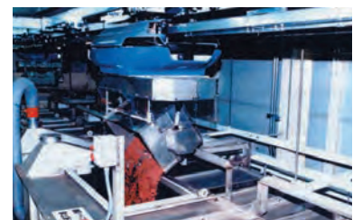
Raw material conveyor system
