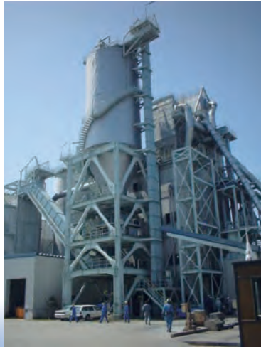
① Bucket Elevator (Tsubakimoto Bulk Systems)
