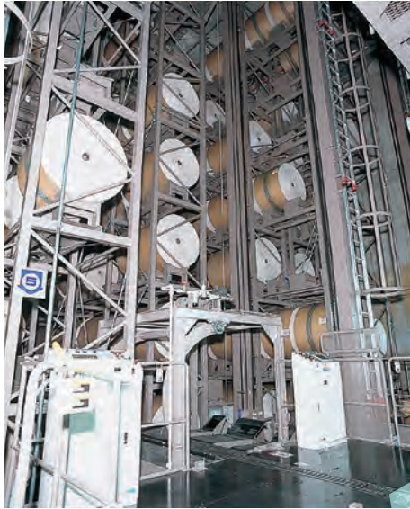
Vertical paper roll storage system
